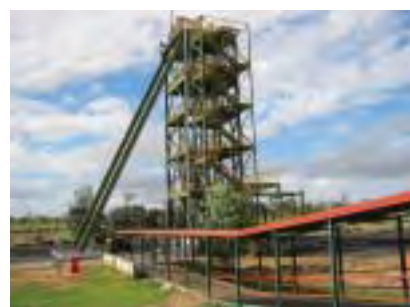
Underground mining (headframe)
